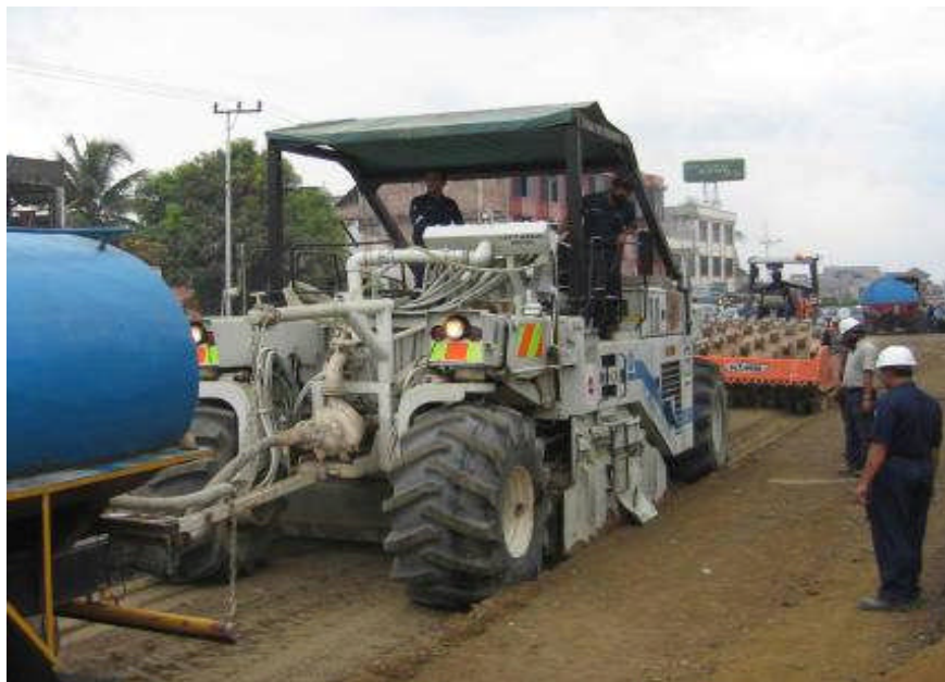
Gambar D.4 - Pencampuran basah ( wet mixing )
