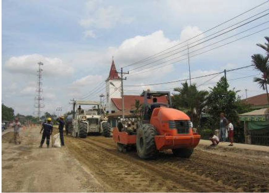
Gambar D.5 - Pematatan awal ( initial compaction )
