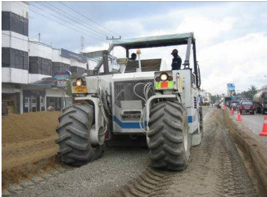
Gambar D.3 - Pencampuran kering ( dry mixing )
